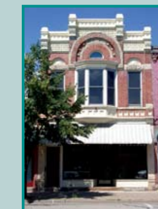
Verkins Building 214 E. Third St. Built: 1890s NR: 1998 This striking building features an elaborate, ornamental, stamped-iron cornice.
