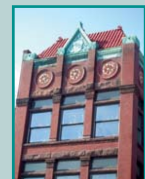
J.A. Merigold and Co. Dry Goods 59 W. Third St. Built: ca. 1868 NR: 1998 Stone rosettes and a stamped copper cornice ornament this three-story brick building.
