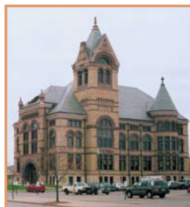
Winona County Courthouse 171 W. 3rd St. Built: 1888 NR: 1970 Architect: Maybury & Son A Richardsonian Romanesque landmark in Minnesota. Winona carpenters, stone masons, and iron workers used regional buff-colored sandstone with trim in Lake Superior brownstone. The main tower rises 136 feet.
